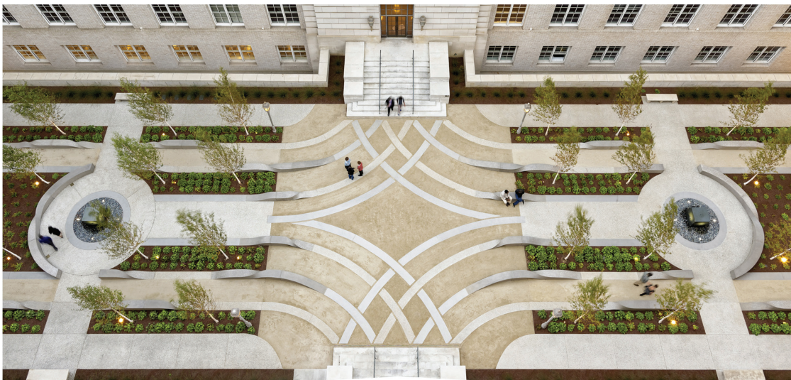
San Francisco general contractor Hathaway Dinwiddie poured ribbons of pavement that define pervious walkways made with decomposed granite.
