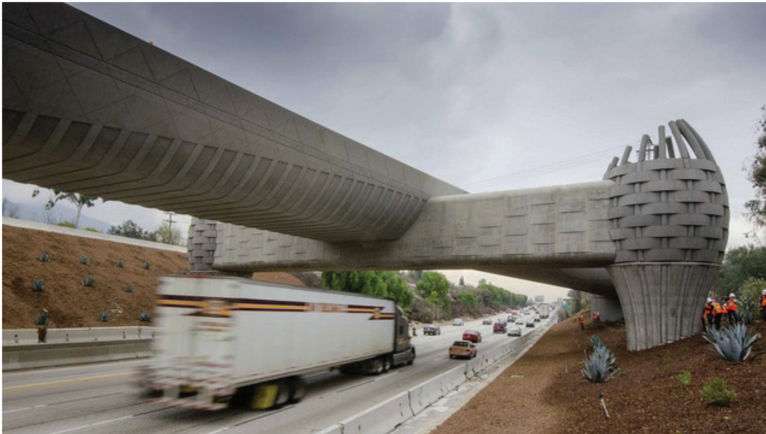
The Gold Line "basket bridge" on the 210 Freeway near Arcadia. (Courtesy Metro LA)
